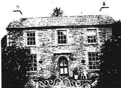
*Facing the green, the south range of Anneth Lowan is a 19th century extension to an earlier, probably 18th century, house. Stucco render has been stripped away to reveal its rubble construction with local Polyphant stone used for dressings over the door and around the windows. The roof is of rag slate, laid in varying widths and diminishing courses. The three over six paned sash windows are an unusual feature of the first floor.*
